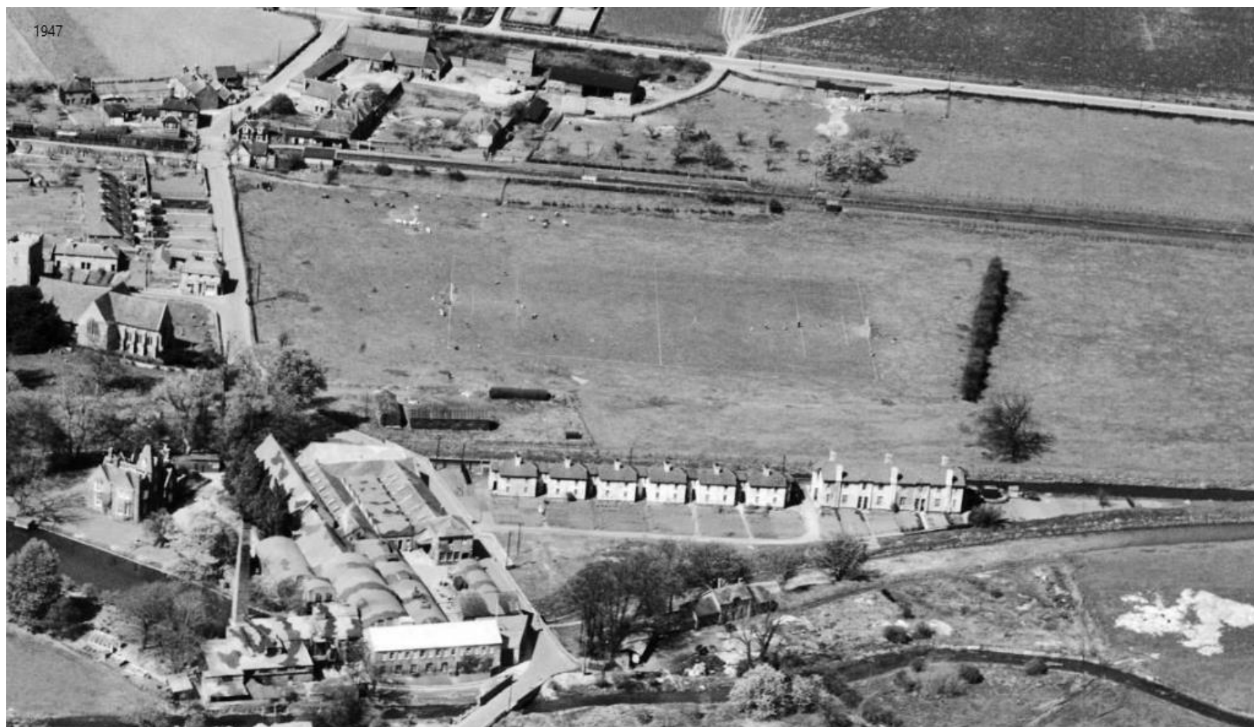
Plate 8: View of the PDA 1947 (facing NNW).
