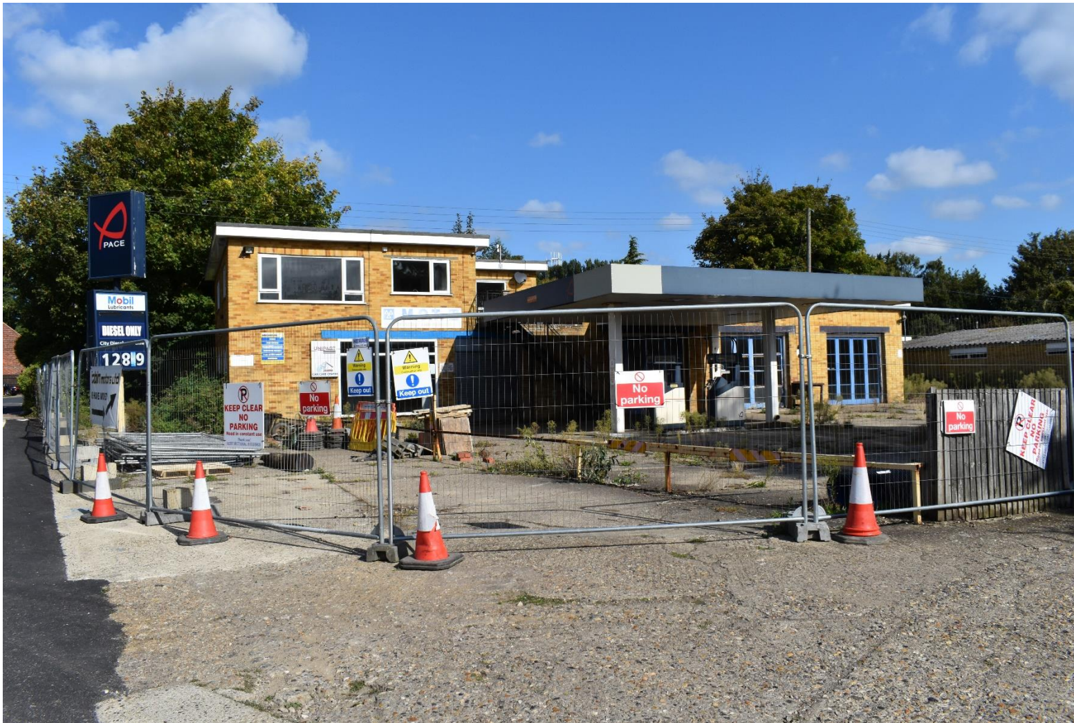
Plate 9: View across the western PDA (facing N).
